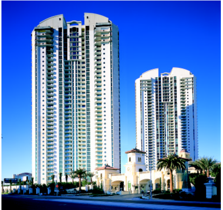
Turnberry Place is the address for elegant, upscale living in Las Vegas with floor plans ranging from 1,550 to 8,000 square feet and prices from $500,000 to more than $5.25 million.
