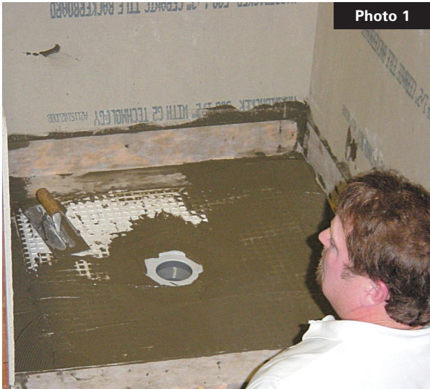
Shown here is an example of an expanded polystyrene shower base used in lieu of the conventional mortar system.
