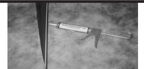
Figura 4. Aplicar NobleSealant 150 (section 6.2).
