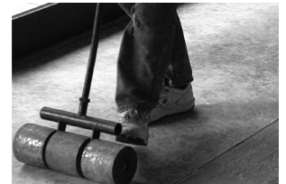
Figura 3. Embeber el Noble Deck (section 5.4).
